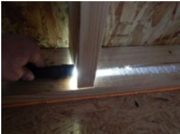
Framing was not properly installed at various areas.
