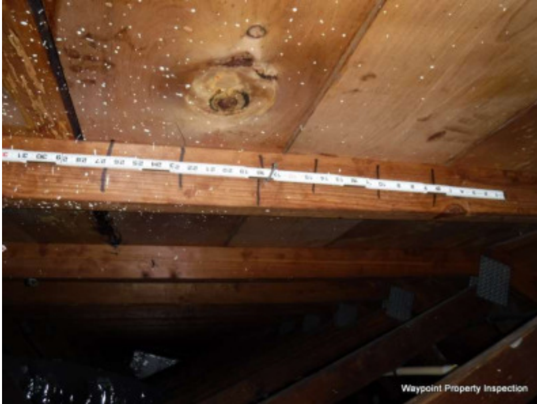
8D Nails, 3 nails per board
