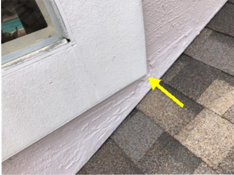
Settlement cracks up to 1/8" inches were visible.
