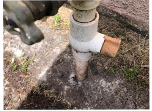
Sprinkler water control valve was damaged/leaking.
