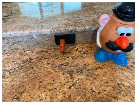
Outlet(s) tested as having reverse polarity at kitchen
