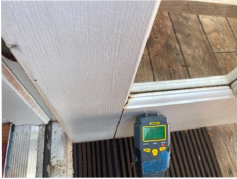
Moisture damage was visible at the secondary door(s).
