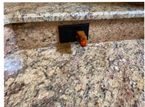
Outlet(s) tested not properly grounded kitchen
