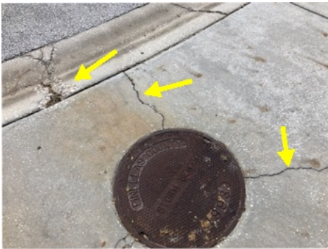
Driveway had large crack(s) visible.
