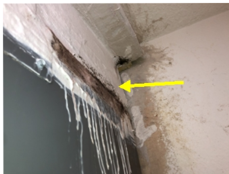
Microbial-like growth was visible at the exterior of the heating unit.
