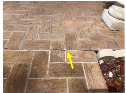
Walkway had large and displaced crack(s) visible.
