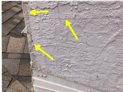
Large and/or displaced cracks were visible at chimney.
