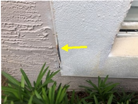
Moisture stains and damage were visible.
