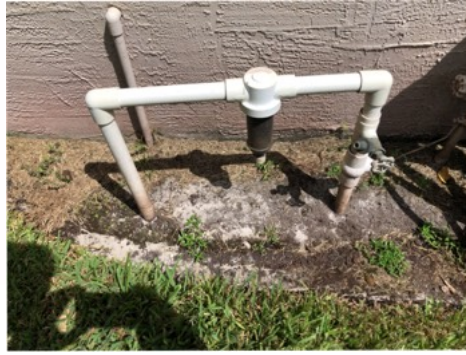
Back-flow valve was not installed.
