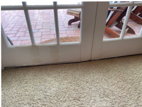
Moisture damage was visible at the secondary door(s).
