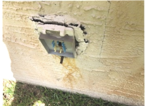
Moisture stains and damage were visible.
