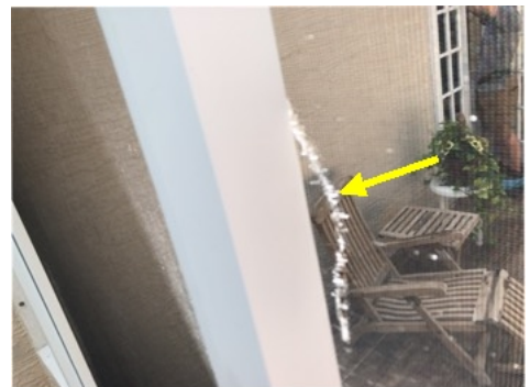
Patio cover screening had visible tears/holes.
