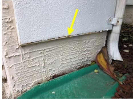
Moisture stains and damage were visible.
