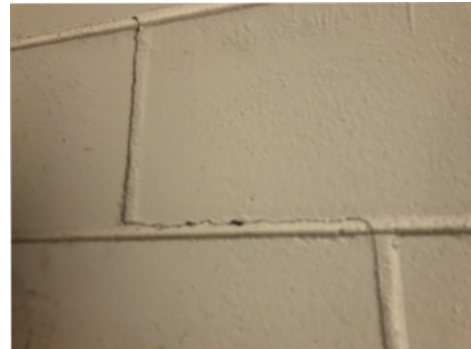
Settlement cracks up to 1/8" inches were visible.
