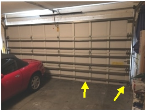
Weatherstripping was deteriorated/damaged and should be replaced.
