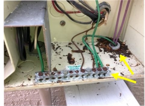
Corroded/damaged buss bar was visible.
