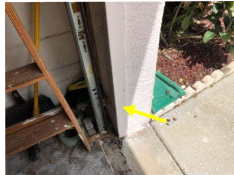
Vehicle door weatherstripping was not installed.
