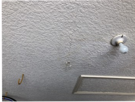
Ceiling finish was worn/deteriorated.
