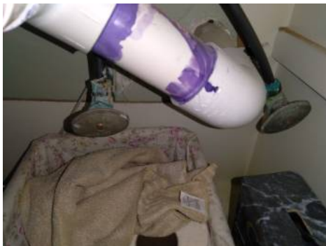
Minor corrosion was visible at the supply lines at master bathroom.
