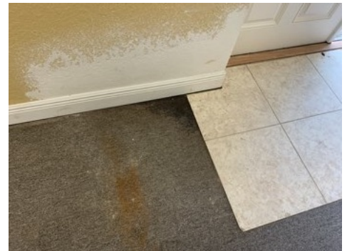
Flooring had visible moisture stains/damage. Stains/damage tested wet using moisture meter.
