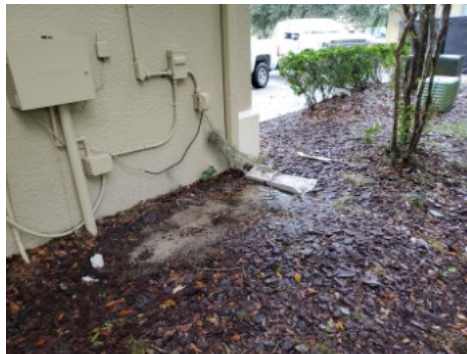
Downspouts should be routed away from the structure for proper draining.
