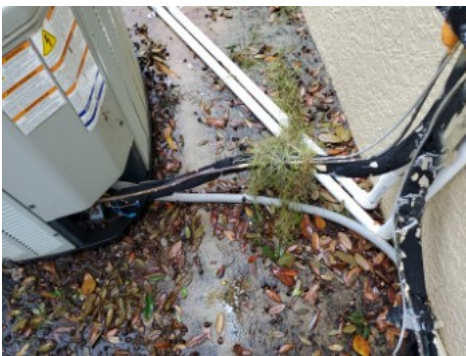
The insulation on refrigerant line was deteriorated.
