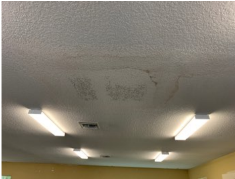
Although dry at the time of the inspection, the visible stain(s) indicated active leaks may be present.
