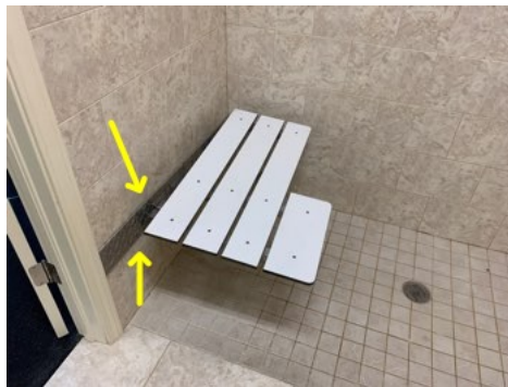
Bench was damaged/not properly secured at men's bathroom left.
