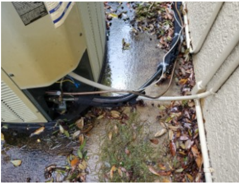
The insulation on refrigerant line was deteriorated.
