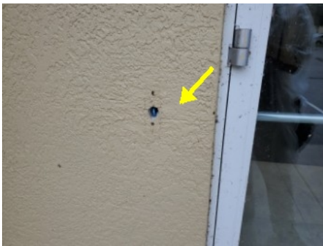
Doorbell was damaged/not installed
