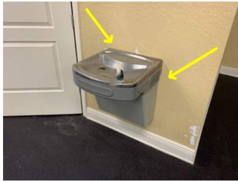
Water fountain was not properly secured to wall.
