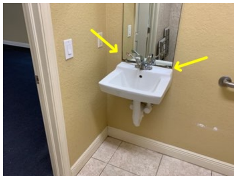
Sink was not properly secured to wall at women's bathroom left.
