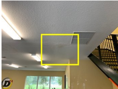
Moisture damage was visible.
