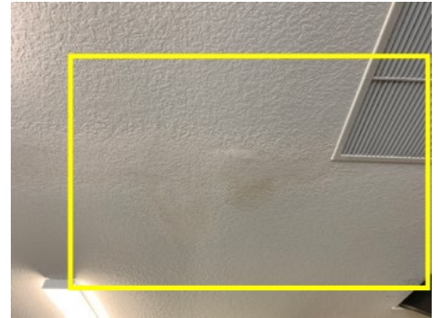
Moisture damage was visible.
