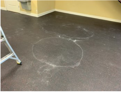
Flooring had visible moisture stains/damage. Stains/damage tested wet using moisture meter.
