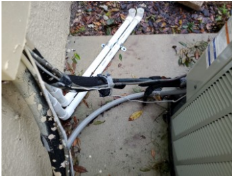
The insulation on refrigerant line was deteriorated.
