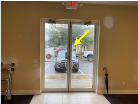
Weather-stripping did not properly seal the front door. Gap was visible.
