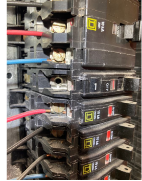
Defective breaker(s) were present.
