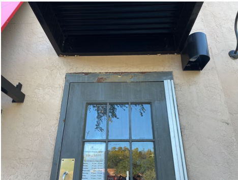
The right side secondary door(s) frame was damaged.
