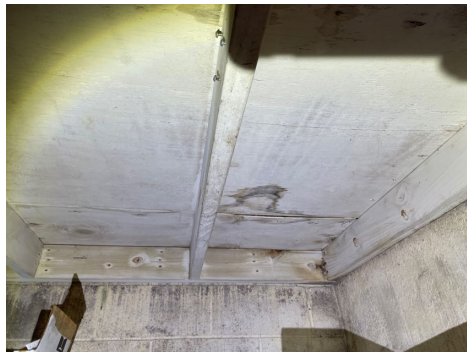
Damaged/deteriorated roof covering was visible.
