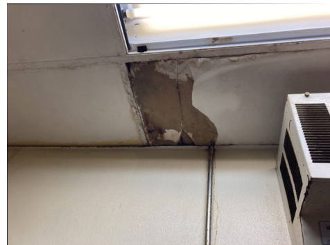
Although dry at the time of the inspection, the visible stain(s) indicated active leaks may be present.
