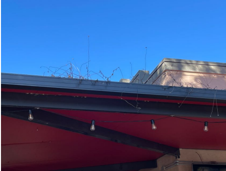
Gutters were filled with debris and the drains were blocked.
