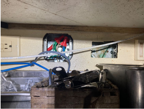
Cover plate(s) were not installed.
