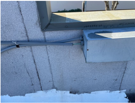
Exposed wiring was not properly protected at various areas of the roof.
