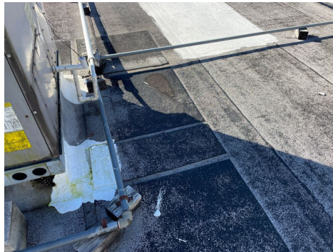
Roof decking had soft spot detected near multiple HVAC systems.
