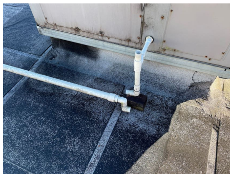
Condensate line was disconnected.
