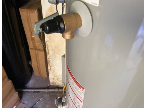
TPR piping was missing.
