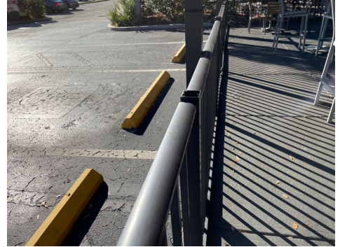
Fence post cap(s) were missing.
