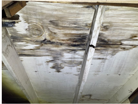
Damaged/deteriorated roof covering was visible.
