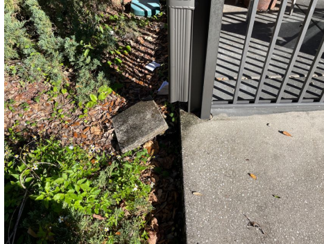
Downspout(s) were missing/not installed.
