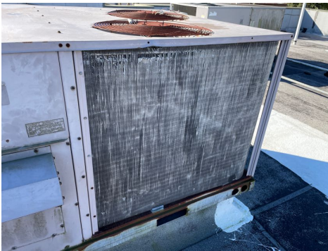
Cooling system was deteriorated.
