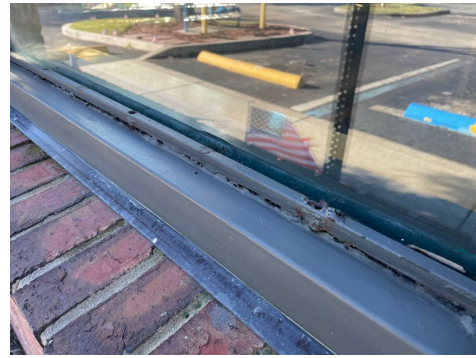
Window(s) frames were deteriorated/damaged.
