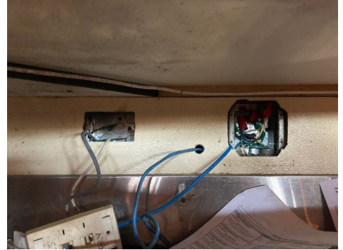
Cover plate(s) were not installed.
