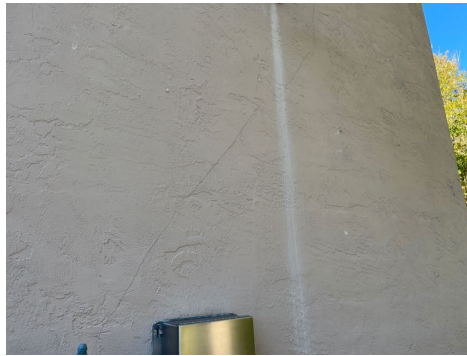
Settlement cracks were visible in various areas.
