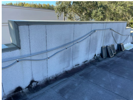
Conduit was not properly secured at multiple locations of the roof.
