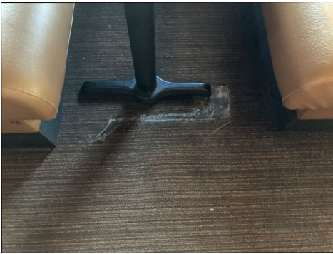
Carpet was worn/deteriorated at high traffic areas.
