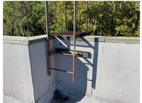
Roof access ladder was loose.
