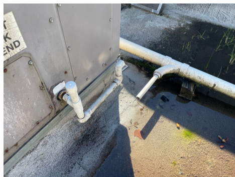
Condensate line was disconnected.
