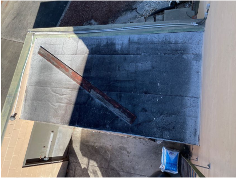
Damaged/deteriorated roof covering was visible.
