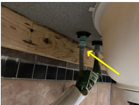
Minor corrosion was visible at the supply lines.
