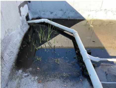
Improper drainage was visible at the rear section of roofing.
