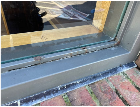
Window(s) frames were deteriorated/damaged.
