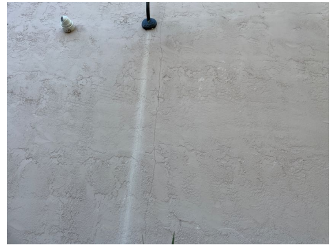
Settlement cracks were visible in various areas.
