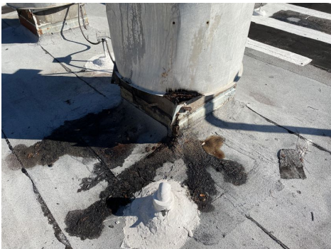
Exhaust hood with grease catch appear to be leaking.
