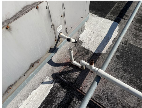
Condensate was disconnected.
