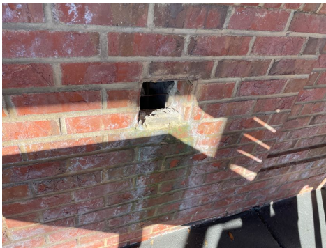
Gaps/holes should be sealed at the front.
