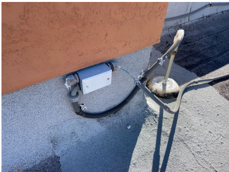
Exposed wiring was not properly protected at various areas of the roof.
