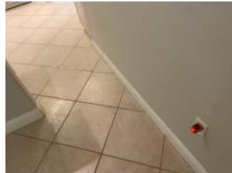
Outlet(s) tested as having improper polarity at interior.
