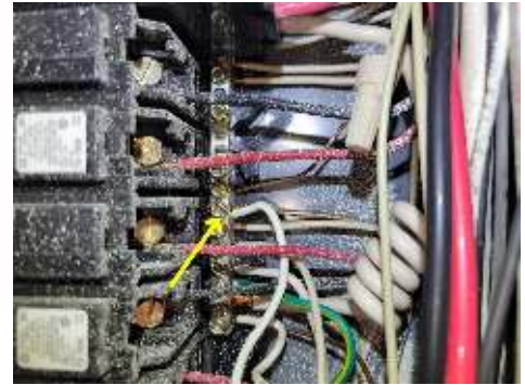
Double Tap connection was visible.
