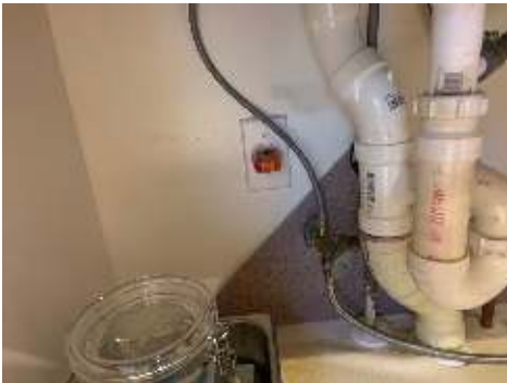
Outlet(s) were not operational at under kitchen sink.
