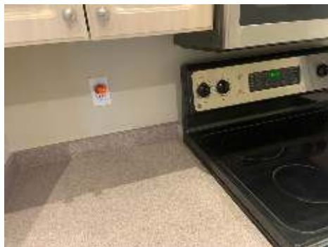
GFCI (Ground Fault Circuit Interrupter) outlet(s) should be installed at kitchen outlets.
