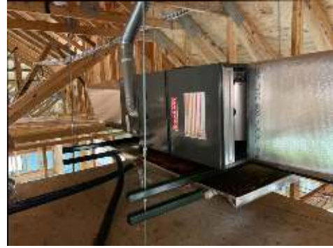
Heating system 1 and 2 were in the process of being installed.
