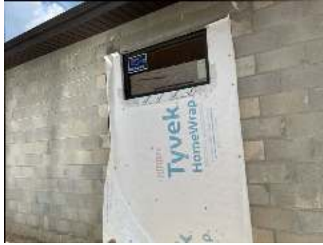
Housewrap/Moisture barrier was installed.
