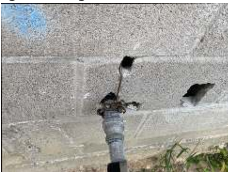
Grounding system was present.
