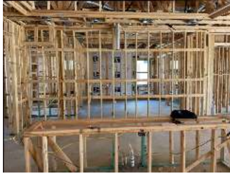
Kitchen sink rough plumbing appeared to be in serviceable condition.
