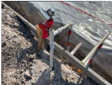
Visible main line rough plumbing appeared to be proper.
