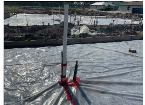
Kitchen supply piping
