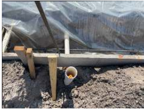
Visible HVAC condensate drain line piping was in good condition.
