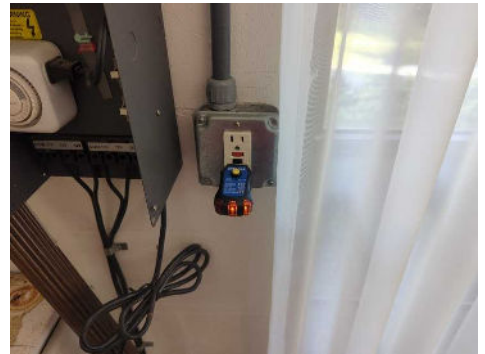
GFCI (Ground Fault Circuit Interrupter) outlet(s) was damaged at garage outlets.
