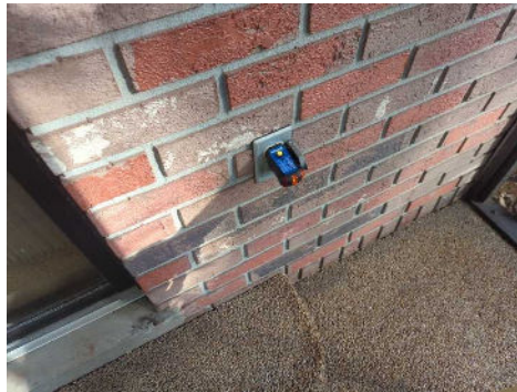
GFCI (Ground Fault Circuit Interrupter) outlet(s) should be installed at all wet areas.
