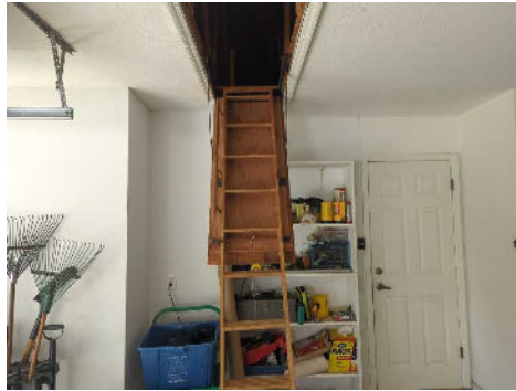
Attic pull down ladder was not fire-rated. (See NACHI Standard of Practice article - https://www.nachi.org/inspecting-residential-attached-garages.htm ).
