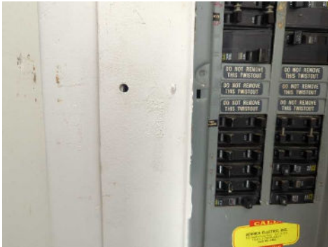
Fasteners were missing.
