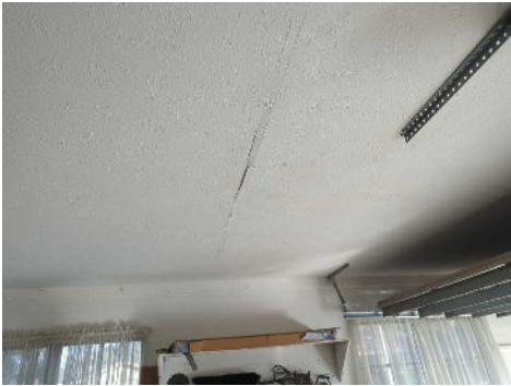
Settlement cracks up to 1/8 inch and/or ceiling seam separation was visible.
