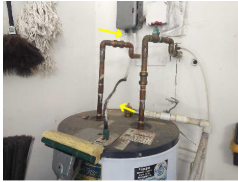
Wiring was exposed visible at water heater.
