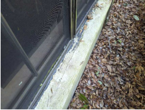
Settlement up to 1/8" cracks were visible at front.
