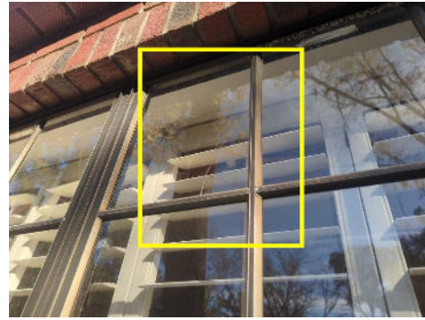
Cracked/damaged glass was present at primary bedroom.
