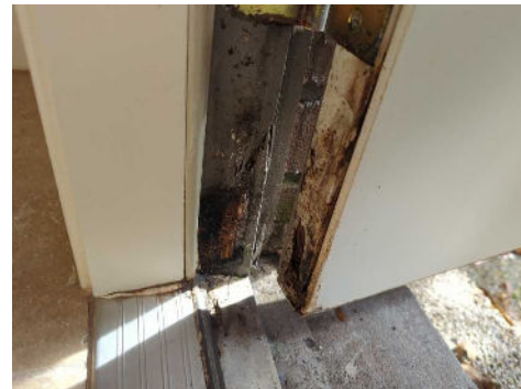
The secondary door(s) had visible moisture damage.
