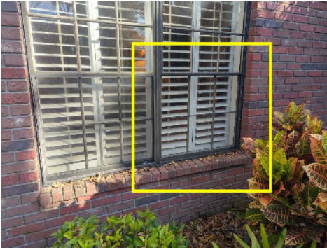
Screen(s) were missing/not installed.
