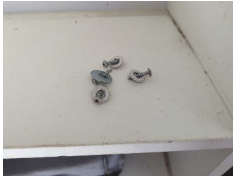
Fasteners were missing and improper.
