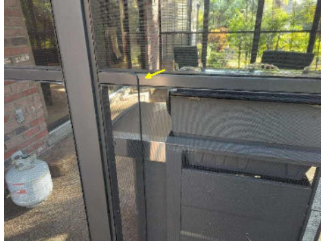
Patio screening was loose/not secured.
