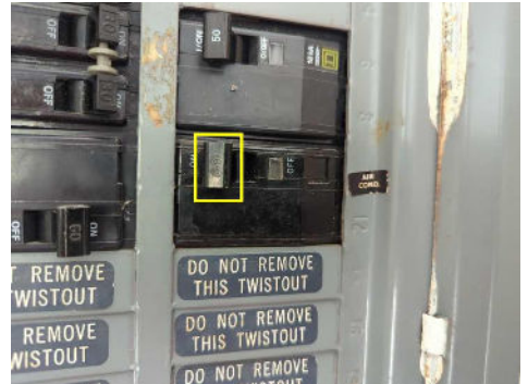
Breaker size at panel exceed the max rating (over fused) at the AC Condenser Unit
