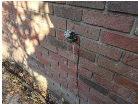
Back-flow device was not installed at the exterior faucets.
